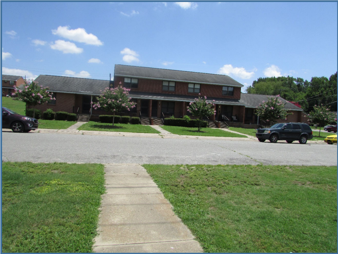
Figure 7. Woodcrest Apartments, 700-710 Bryant Street, view to the east.
