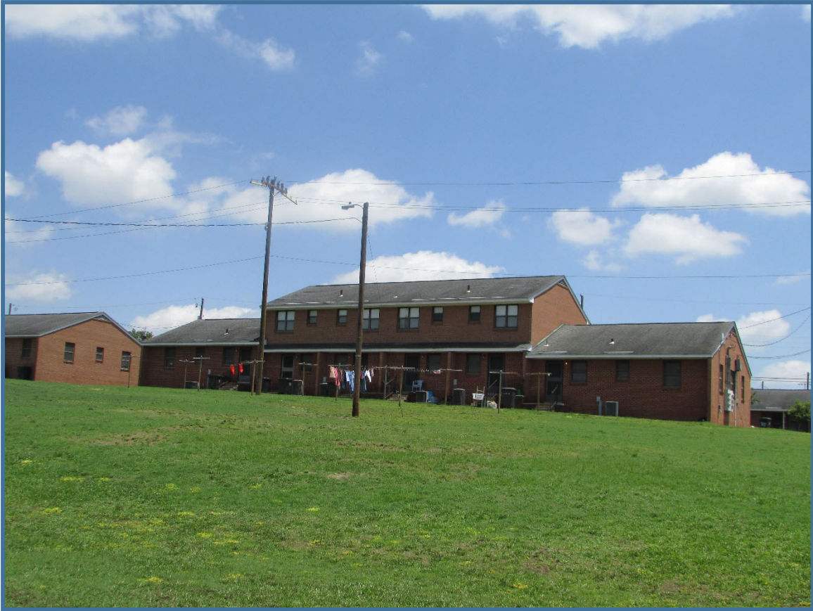
Figure 8. Woodcrest Terrace Apartments, 701-711 Bain Street rear elevation, view to the east.
