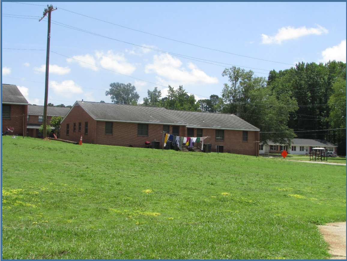
Figure 10. Woodcrest Apartments, 701-703 Bryant Street, view to the southeast.
