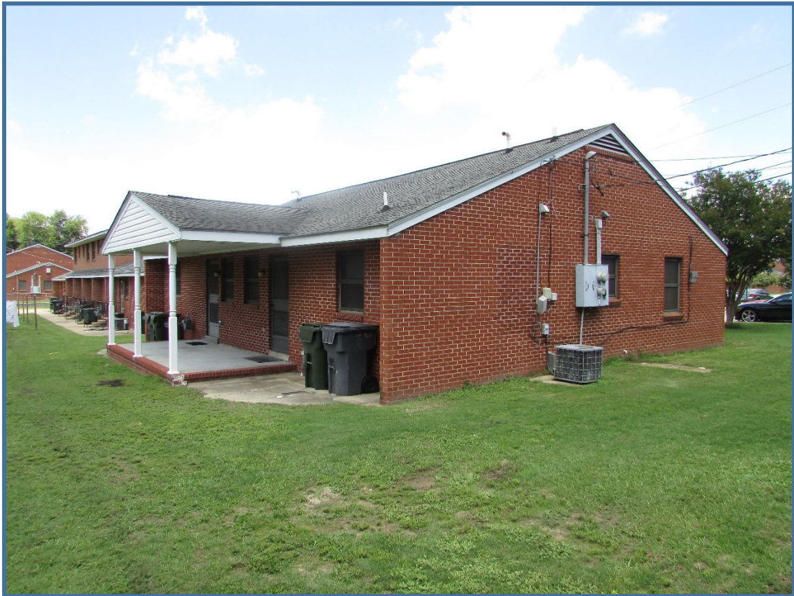
Figure 4 Woodcrest Apartments, 705 Bryant Street, view to the south.
