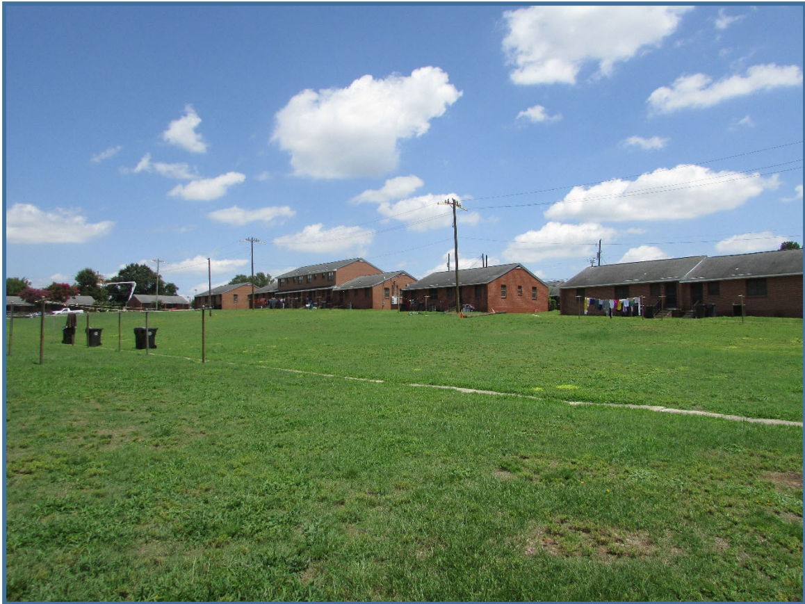
Figure 14. Woodcrest Apartments, 701-719 Bryant Street, rear elevation, view to the northeast.
