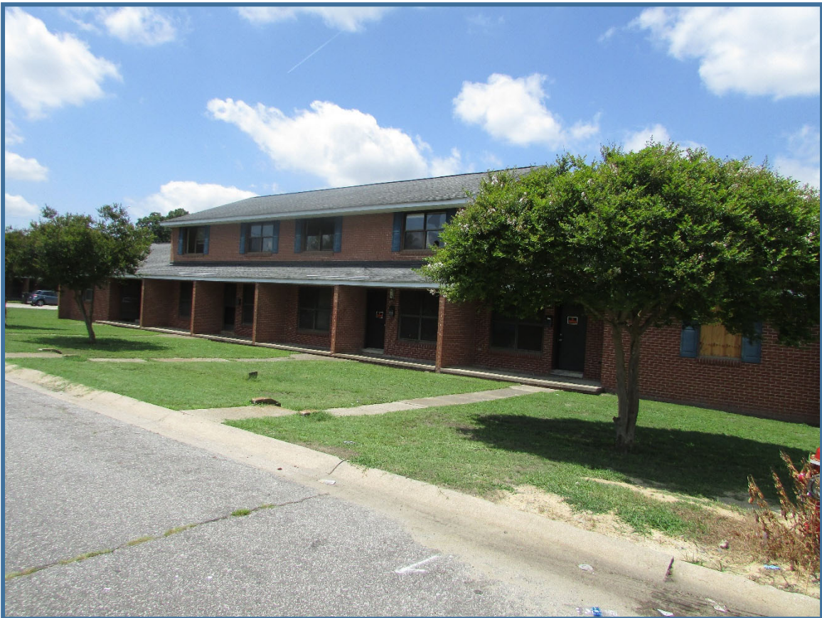
Figure 17. Elmwood Terrace Apartments, Goldsboro, North Carolina.
